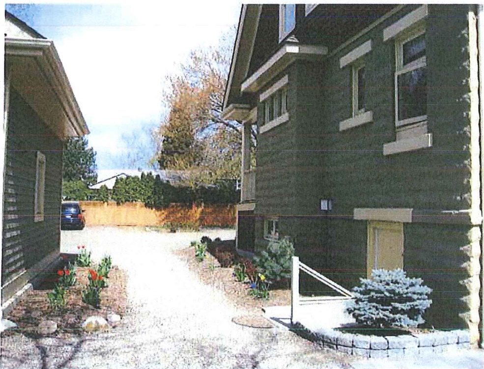
Basement Entrance (one of two)
